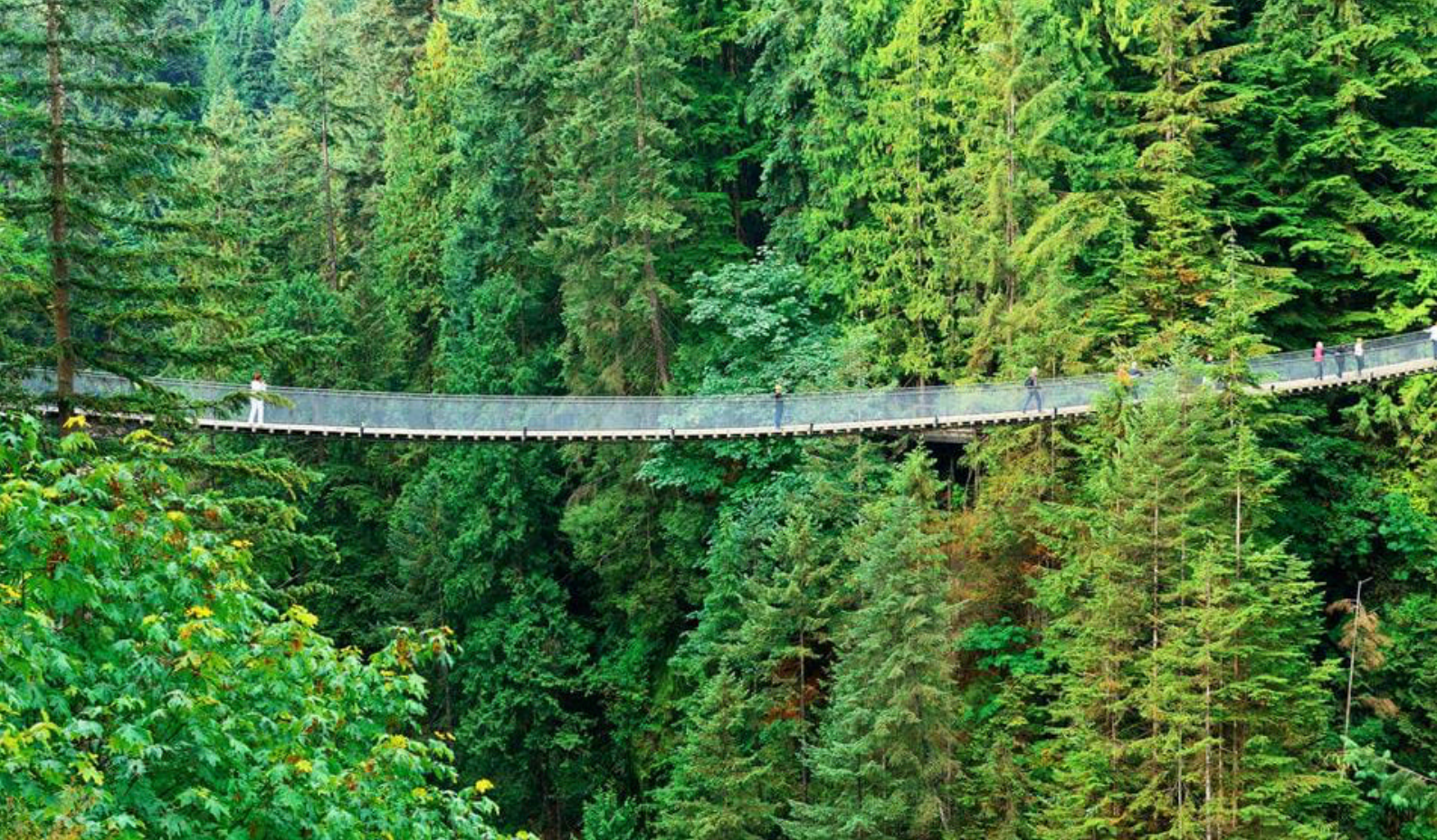
Capilano Suspension Bridge
