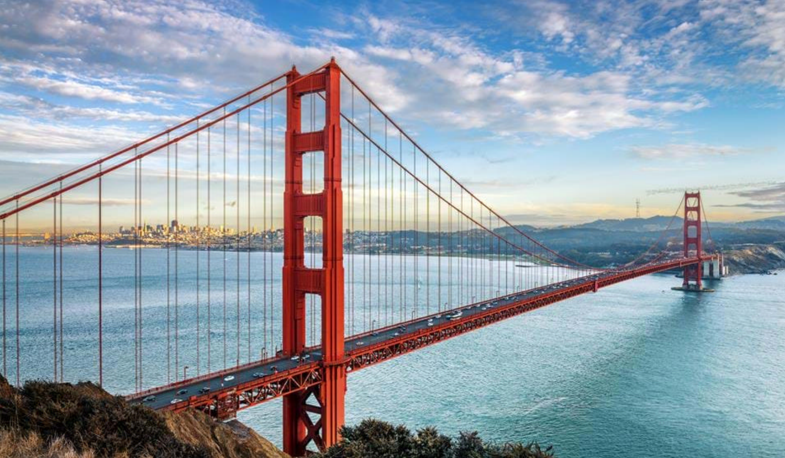
Golden Gate Bridge, San Francisco
