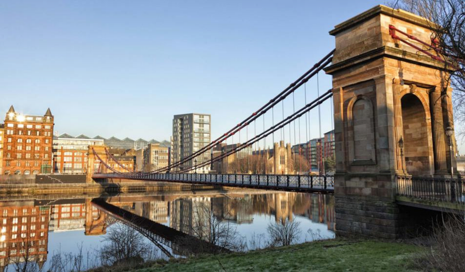
South Portland Street Bridge i Glasgow
